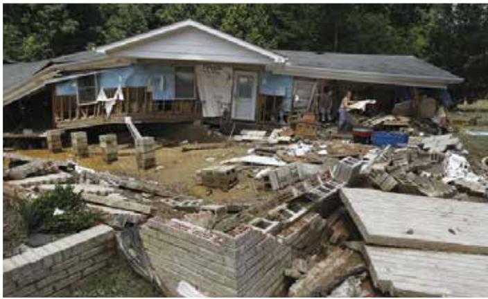
TOP: Flooding in Madison County in May 2010 reduced this roadway to warped sheets of asphalt. INSET: Roaring waters along Harless Creek in Pike County destroyed this residence during a July 2010 flood. OPPOSITE LEFT: A pile of debris is all that remains of this home after flooding in Pike County in May 2010. Photos provided by DOW
